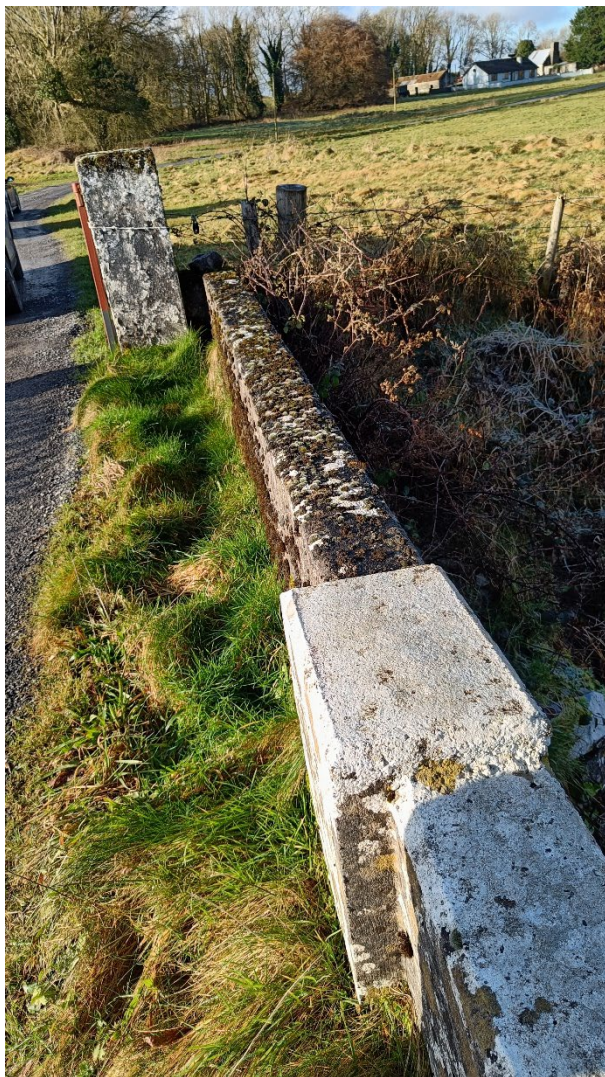
Appendix 5: Northern parapet view facing entrance of property – showing parapet covered in moss.
