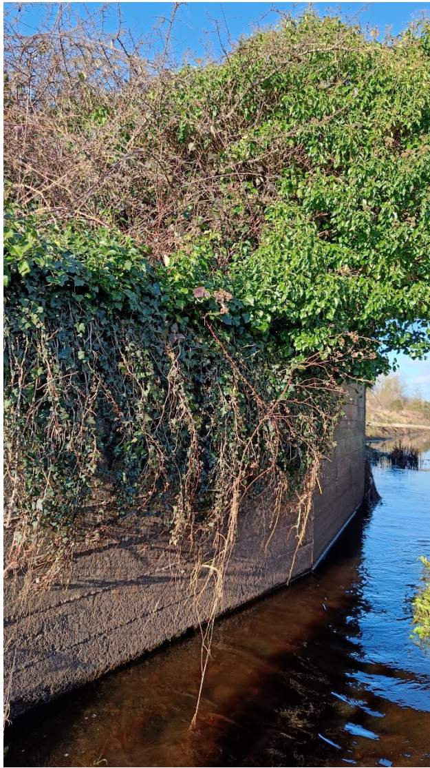
Appendix 10: West abutment view along the southern side – showing heavily vegetated abutment/ soffit of the bridge deck.
