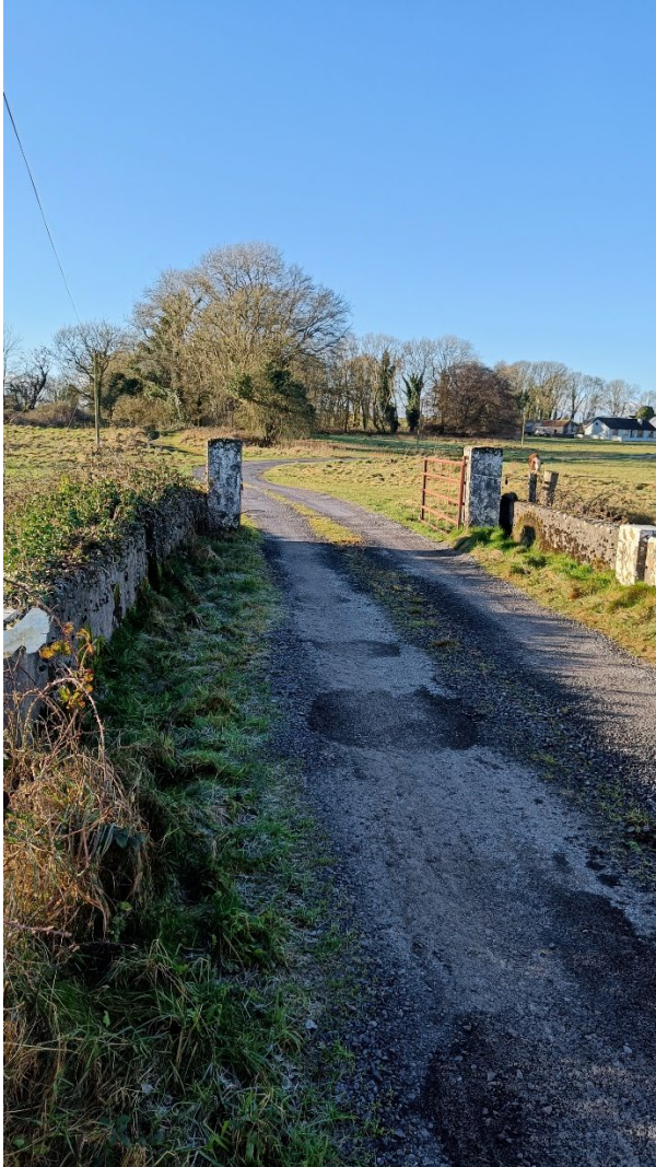
Appendix 1: Road surface: View facing west from the east side of the structure showing minor raveling along the side of the carriageway.
