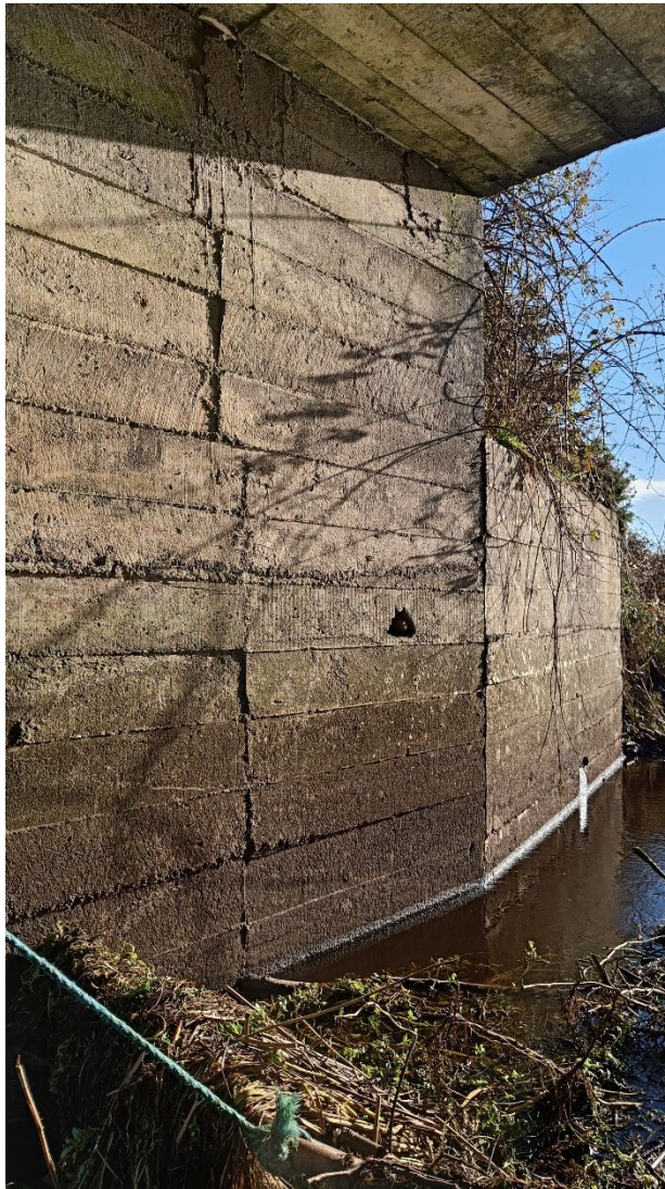
Appendix 12: East abutment view along the northern side – showing 1 no. minor crevices located 1m above the water level and 0.4m from the face of the bridge approximately.
