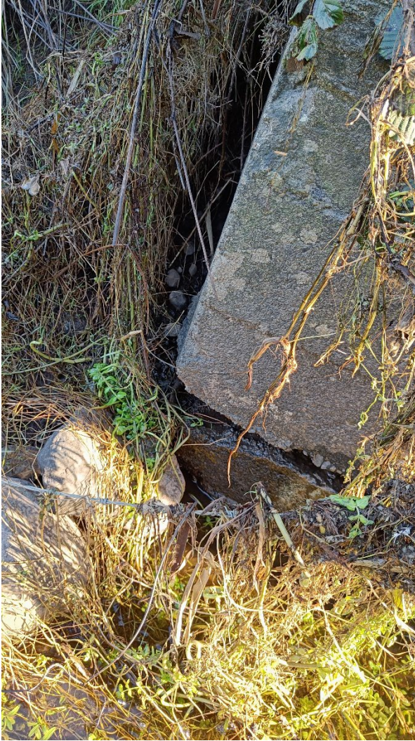
Appendix 20: Crack shown at the East Abutment side wall along the northern side of the bridge.
