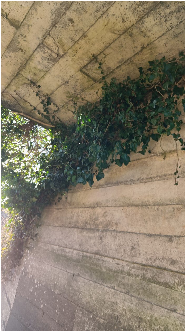
Appendix 14: West abutment and deck soffit front view – showing overgrown vegetation.
