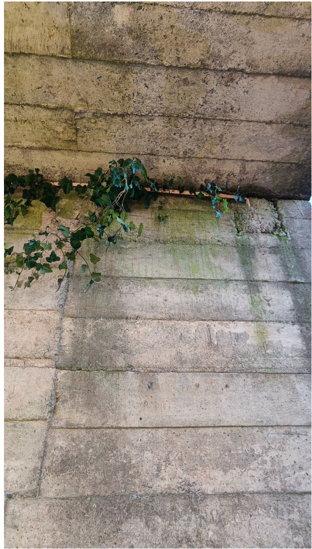
Appendix 15: West abutment and deck soffit front view – showing concrete honeycombs area and overgrown vegetation.
