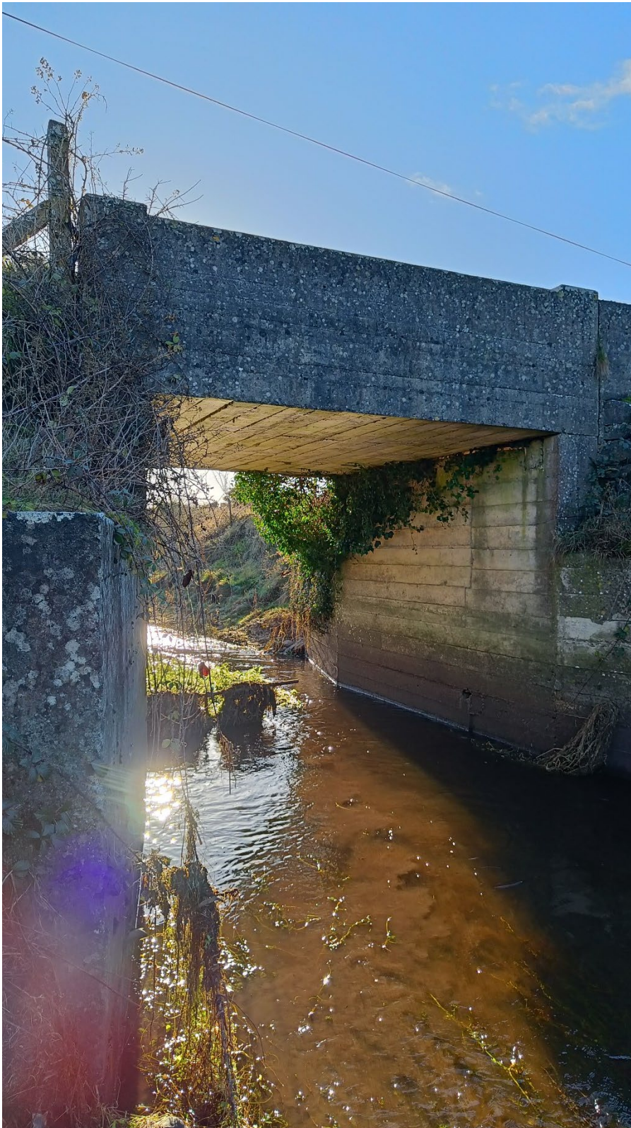
Appendix 7: View of the bridge from riverbed north side – showing heavily vegetated soffit of the bridge deck.
