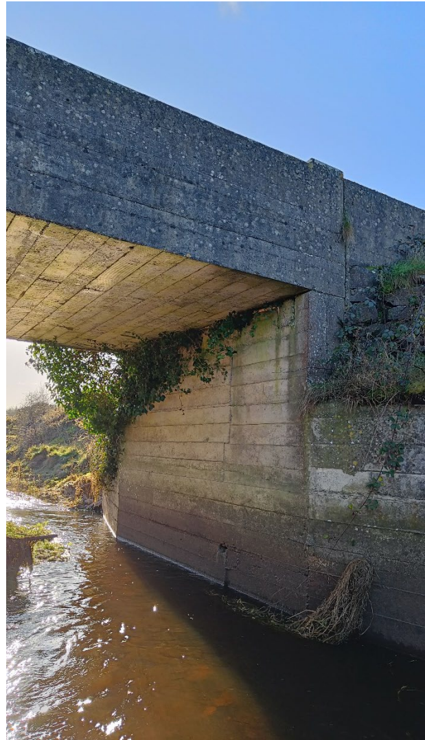
Appendix 9: West abutment view along the northern side – showing heavily vegetated soffit of the bridge deck and minor crevices approximately 0.5m above the water level at the center of the abutment.
