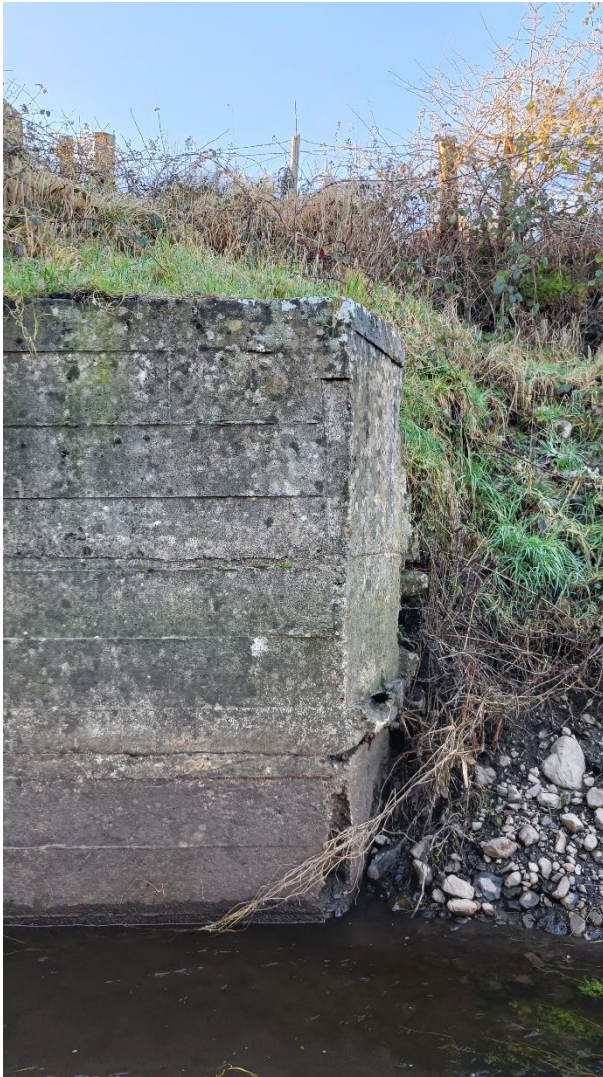
Appendix 8: West abutment view along the northern side – cracks shown at the bottom of the abutments needing repairs.
