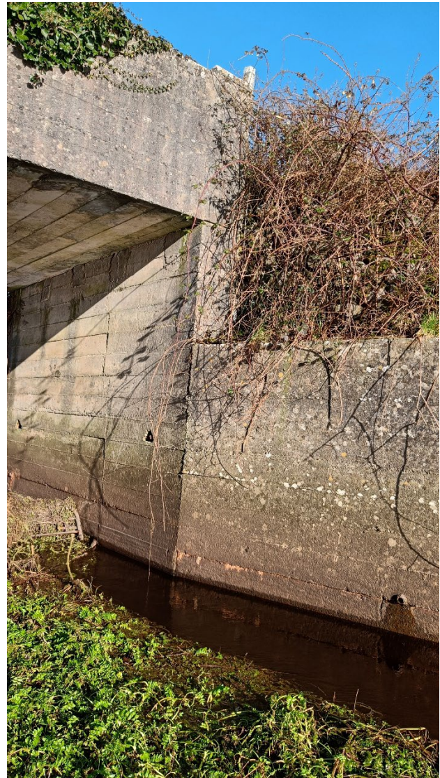
Appendix 11: East abutment view along the southern side – showing 2 no. minor crevices located 1m above the water level and 0.4m from the face of the bridge approximately.
